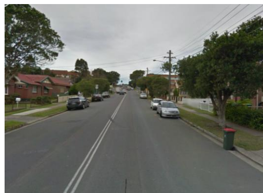
Figure 2.4: Pomeroy Street – Looking East
